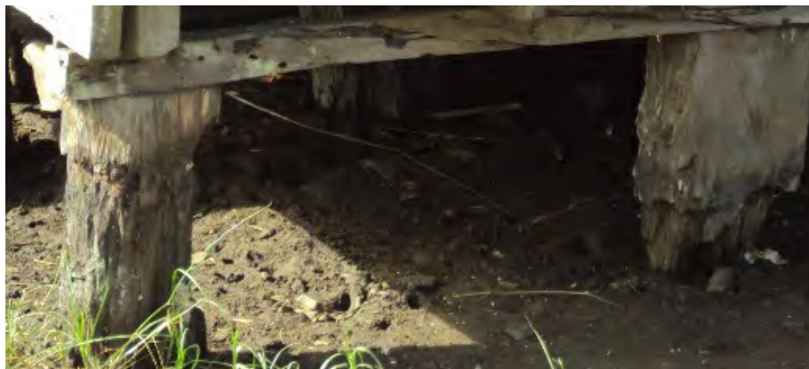
Figure 6. Weathered of wood of the stilts houses
